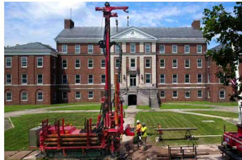
Rotosonic drill near historic hospital extracting continuous core down to 125ft.—through glacial till, original 19th century seawall, to bedrock.
